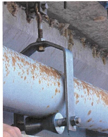
Figure 4: Roller hanger
