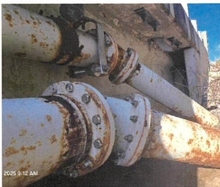
Figure 1: Force main exit location at bridge abutment
