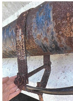
Figure 10: Damaged hanger
