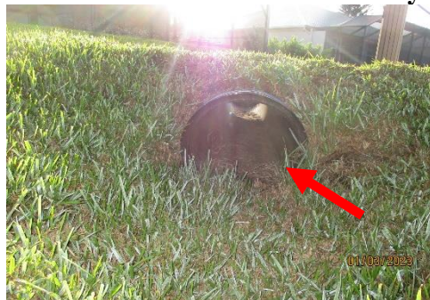
Silt in Culvert at 163 Sunset Cay
