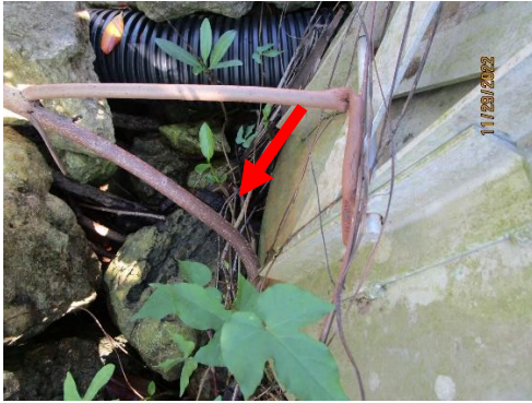
Root Pushing on Flapper
