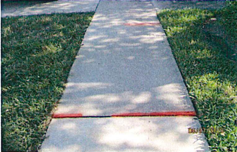
Sidewalk Grinding @ 128 Cays Dr.
