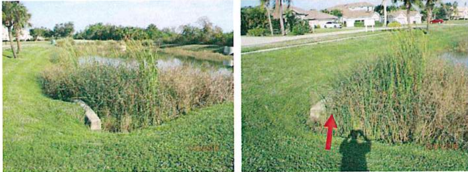
Headwall in Retention Pond #2
