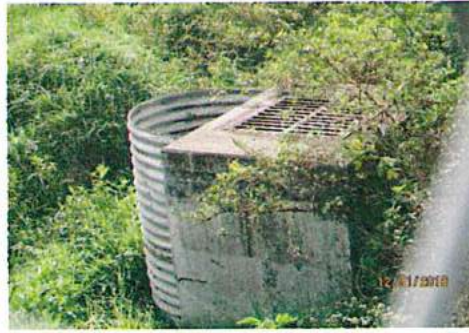
WCS at Water Plant
