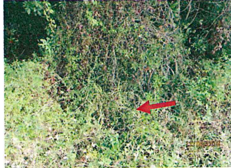
Outflow Pipe behind Vegetation
